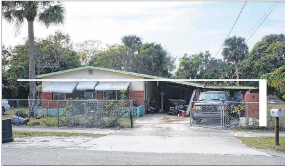
This is the home of Carrie West, 92, who will be getting a new roof on her house as part of a joint effort between Habitat Angel and Keep Martin Beautiful. CONTRIBUTED
